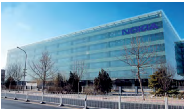
Nokia Headquarters Business Building, Beijing, China
