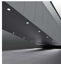
Soffit LED spot cladding lighting
