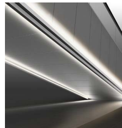
LED cove lighting Side and soffit cladding
